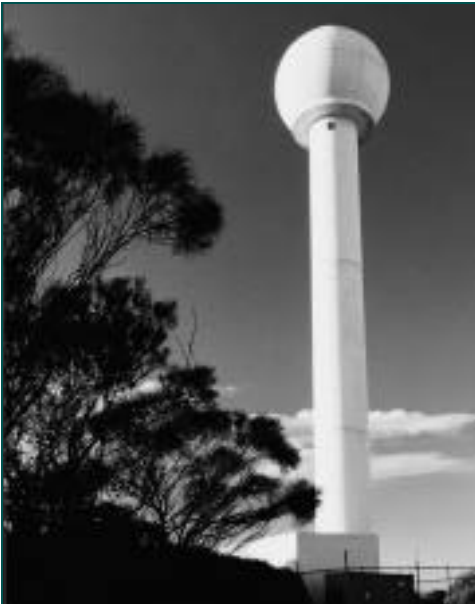
Left Bureau of Meteorology new weather radar at Kurnell, NSW – part of a network of data stations
