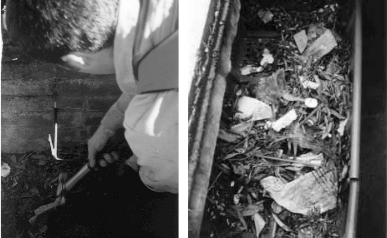
Photograph 5.9 Installing Banyule City Council side entry pit traps in Coburg
