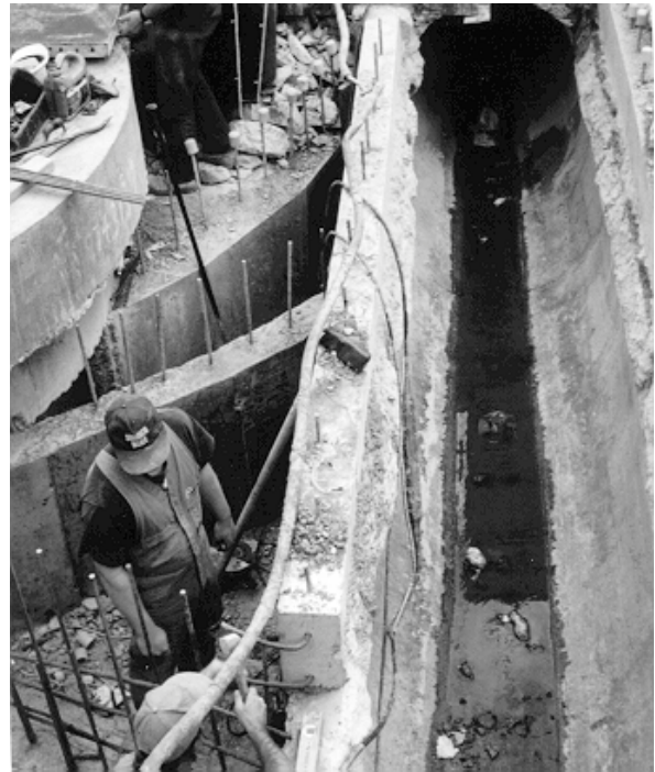
Photograph 5.5 Construction adjacent to the drain
