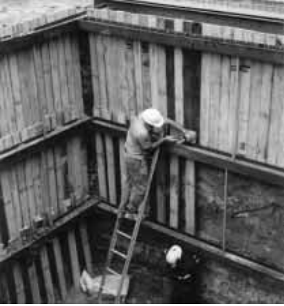
Photograph 5.1 Excavation down to the floor of the chamber,(6x6x4 meters)
