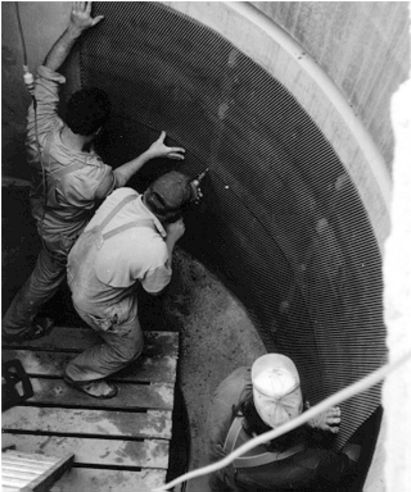
Photograph 5.4 Fitting the separation screens
