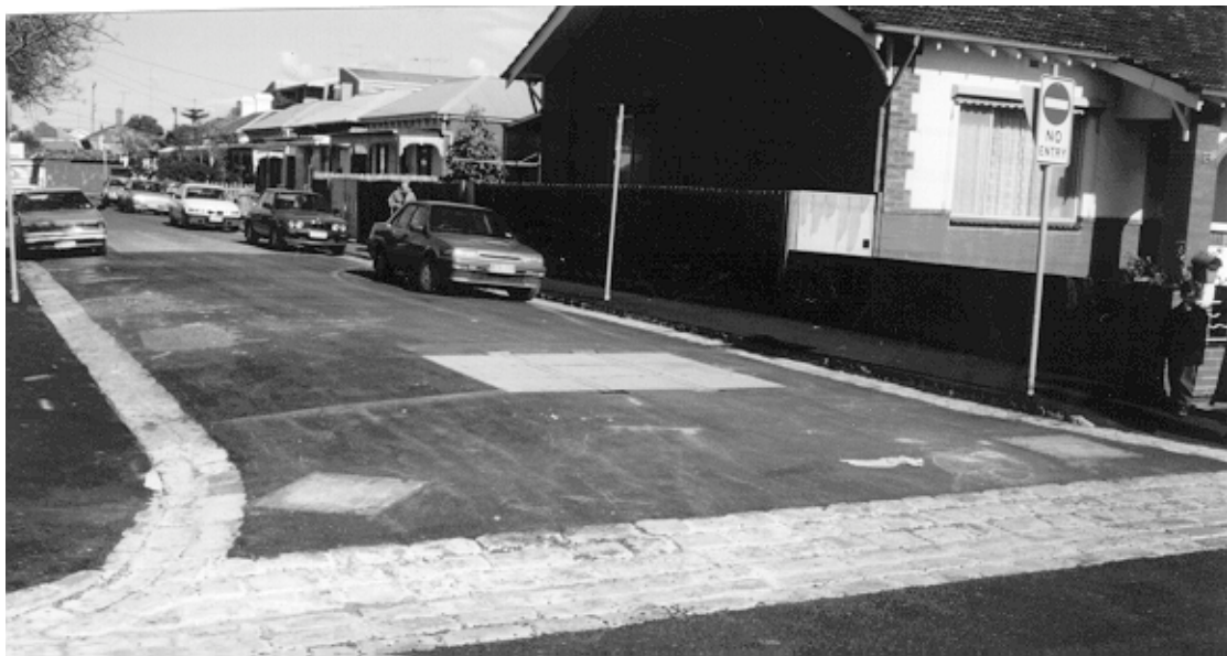
Photograph 5.6 The final product at road level
